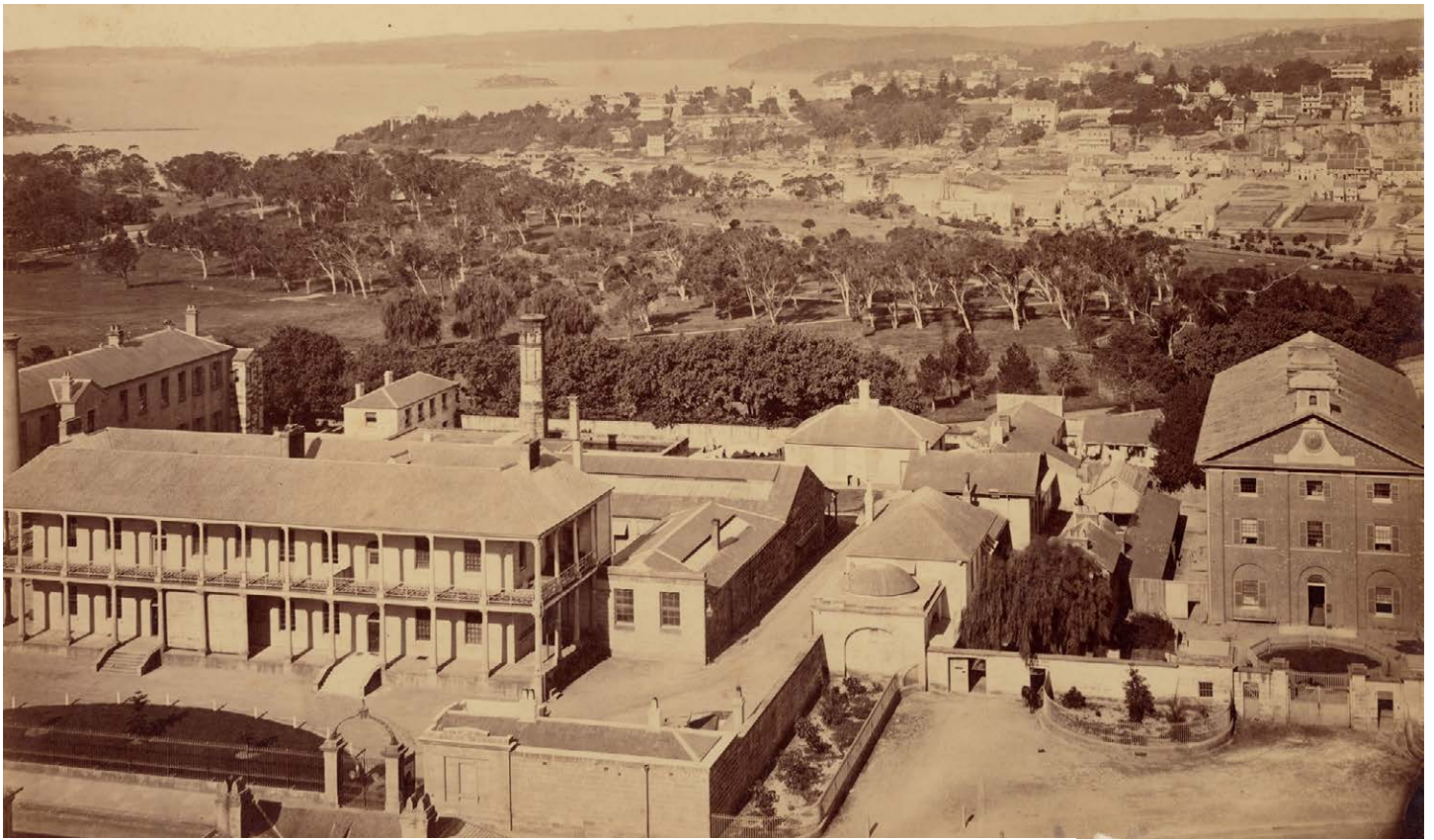
Panoramic view taken from the steeple of St. James Church, 1871 (SLNSW)
