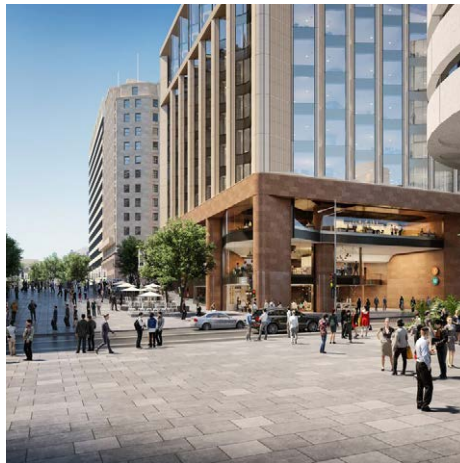
New Martin Place Metro and associated development (Metro Martin Place)
