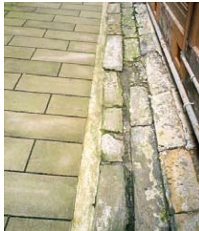
Figure 1.2 Longs Lane. New fabric and old.
