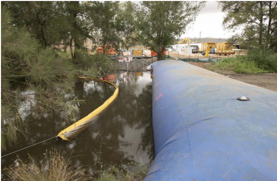
Figure 28. Tamworth temporary weir in 2019 (Bendigo Advertiser)
