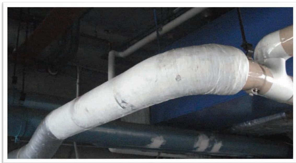
Figure 8 - Friable Asbestos – Pipe lagging
