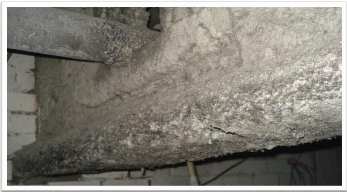
Figure 9 - Friable asbestos – Sprayed fire insulation on beams
