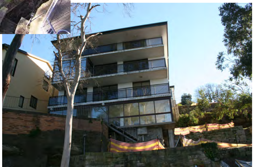
Photo 2. Building on No. 11 Nelson Parade (from the backyard)
