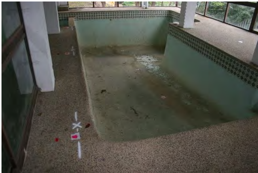
Photo 3. Bore hole locations in pool area of the building
