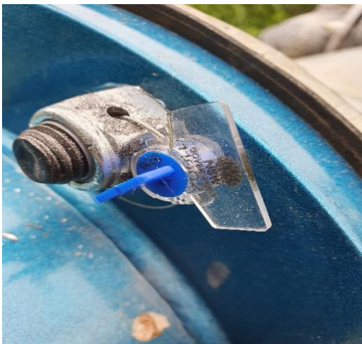
Figure 11. DQP seals on the flange bolt and the flow meter termination enclosure
