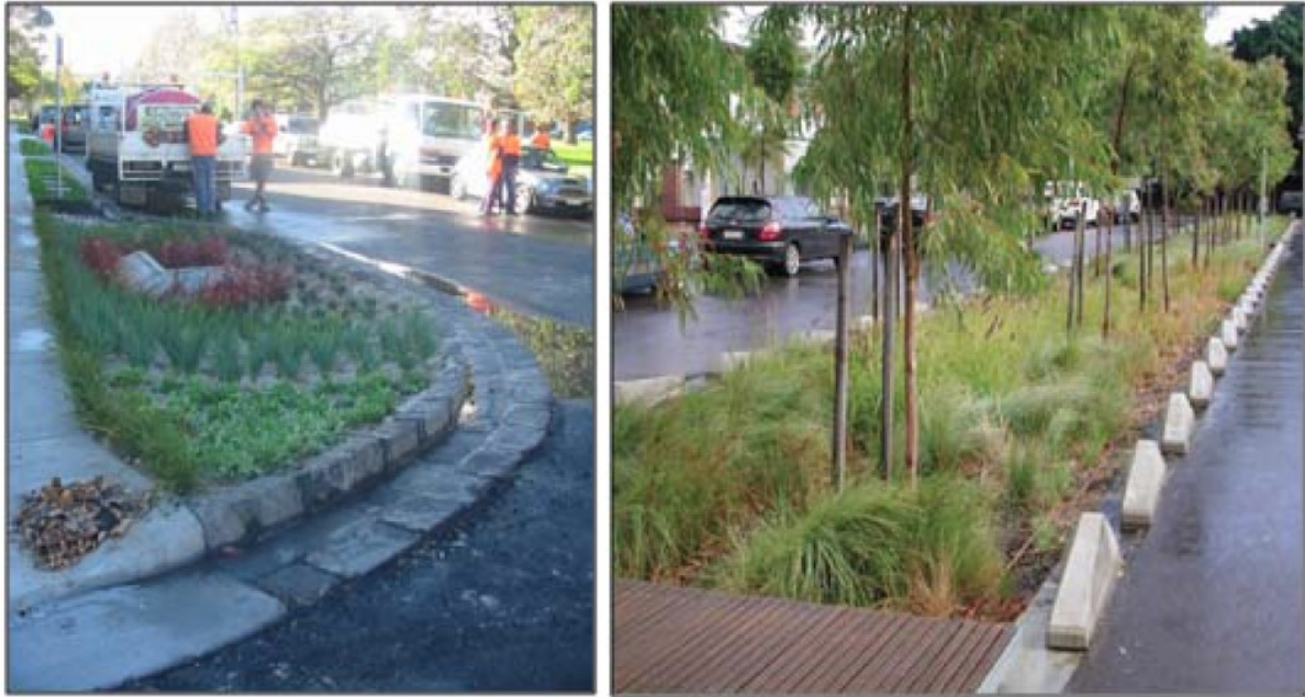
Figure 15. Vegetated filtration systems in swale-type (left) and basin-type (right). Source: Monash University 2010.
