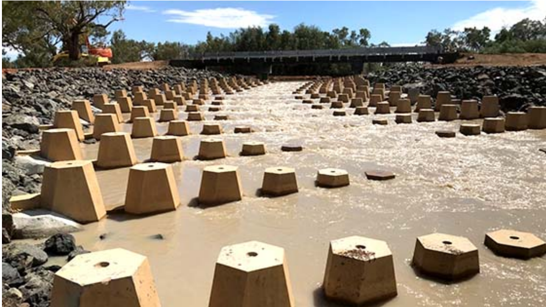
Fish-level perspective of Homestead Fishway, demonstrating a consistent drop in water level that allows fish to easily and quickly ascend upstream or downstream. Credit: Dr Matthew Gordos, DPI Fisheries.
