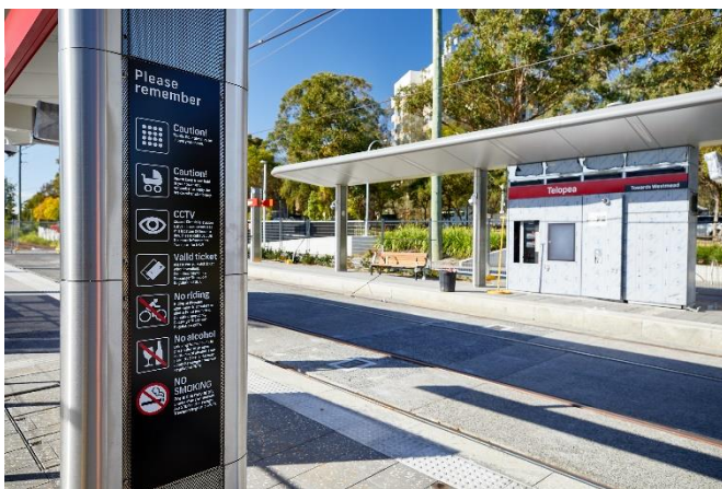
New light rail station at Telopea
