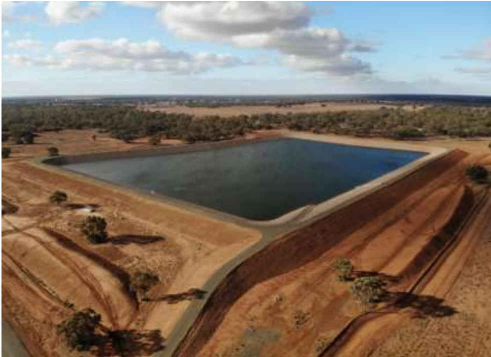
Nyngan offstream storage
