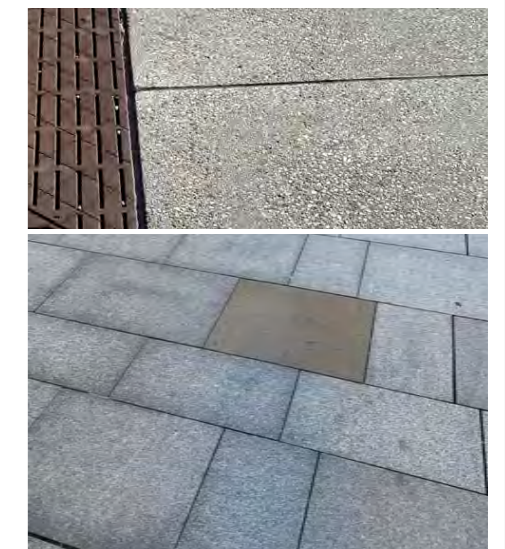
Park Edge Robust and simple materials such as exposed concrete or mixed light coloured stone
