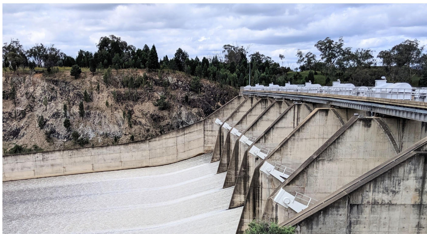
Image courtesy of Ines Richter, Department of Planning and Environment. Burrendong Dam Spillway.
