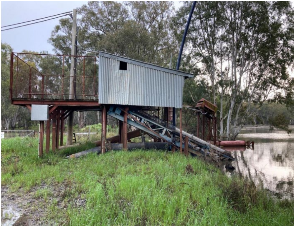
Figure 3 shows the existing Elwah Pump Station on the Murrumbidgee River proposed to be upgraded. Source: Pinion Advisory, 2023.
