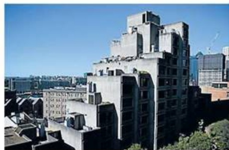
The Sirius building at The Rocks.
