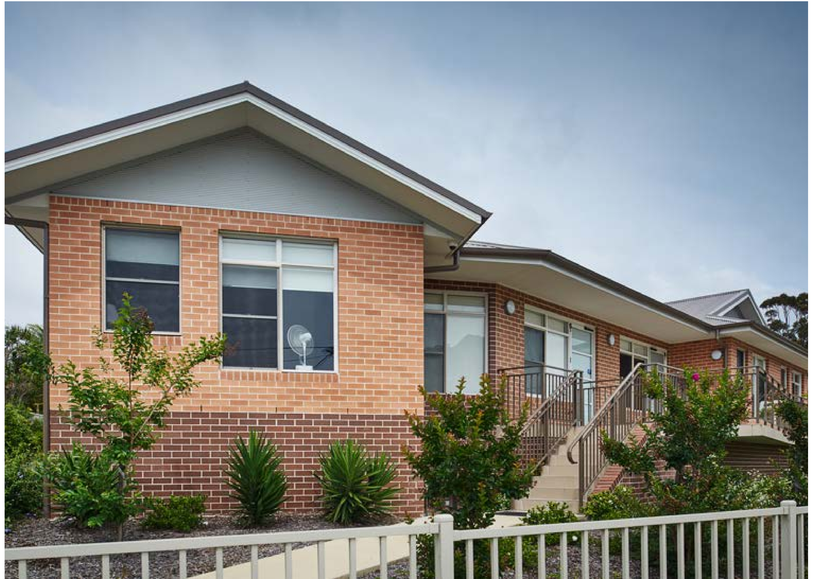
After Social housing in the Northern Beaches LGA – safe, well-designed and appropriate.
