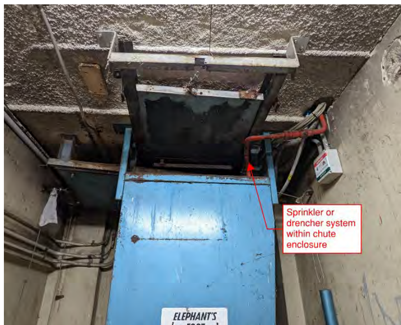
Figure 0-2 - Garbage room chute system - Sprinkler or drencher system.
